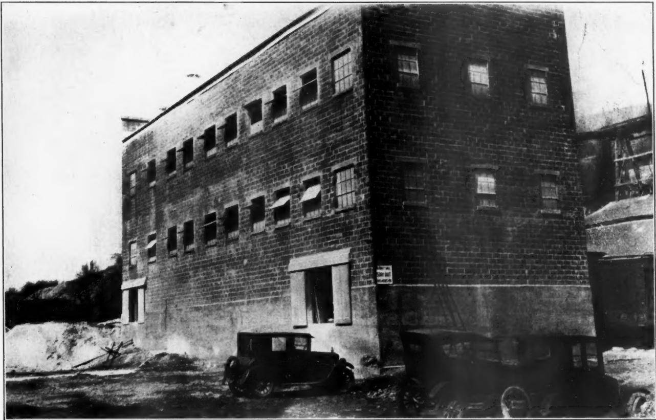
This is the Hydrate Building. The Material is Elevated Vertically and Then Conveyed Horizontally from the Kiln Building at the Right and Discharged Direct to the Hopper of the Hydrator.
